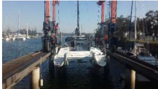
Yamba Marina repairs
